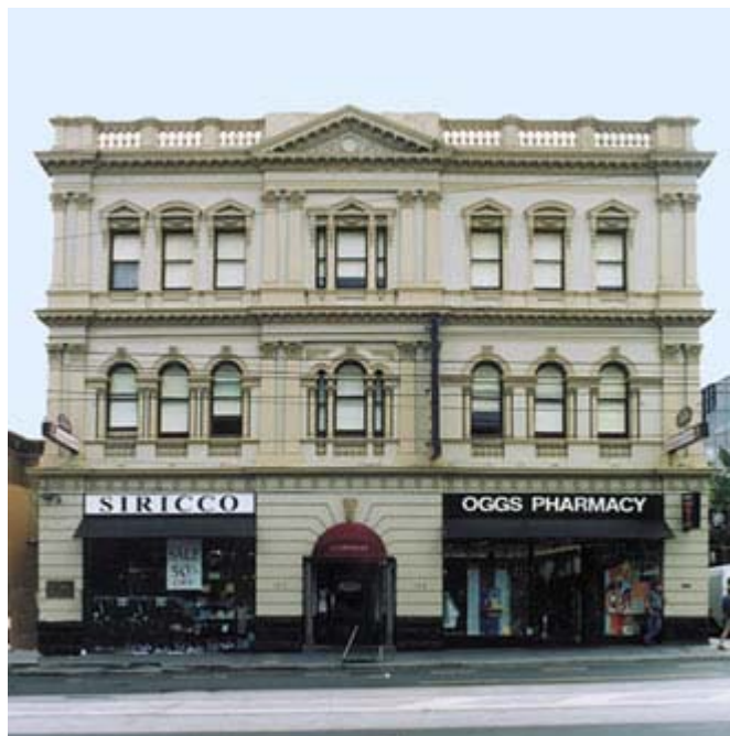
Victorian Style Building in Claremont Cape Town
